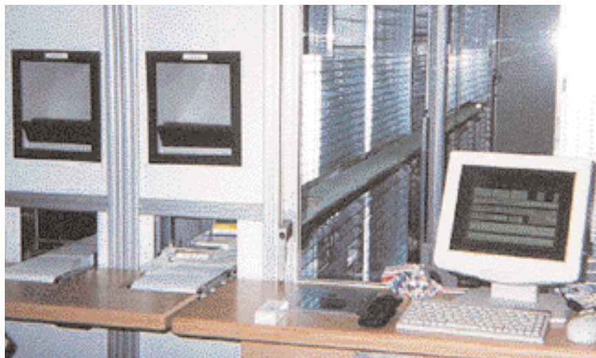
Installing automated dispensing systems can allow pharmacy staff to spend more time on wards
