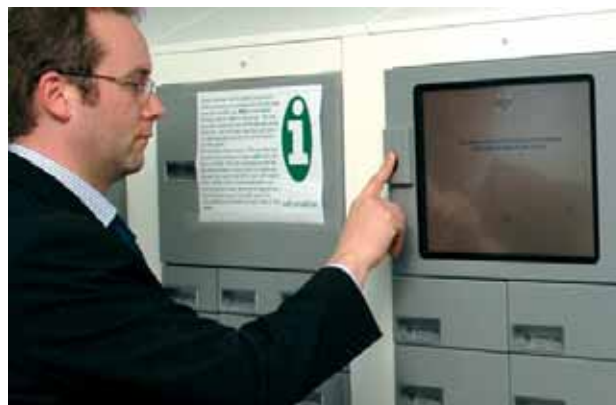
Fingerprint scanners prevent unauthorised access to medicines stored in a ward-based Medi 365 automated dispensing unit
